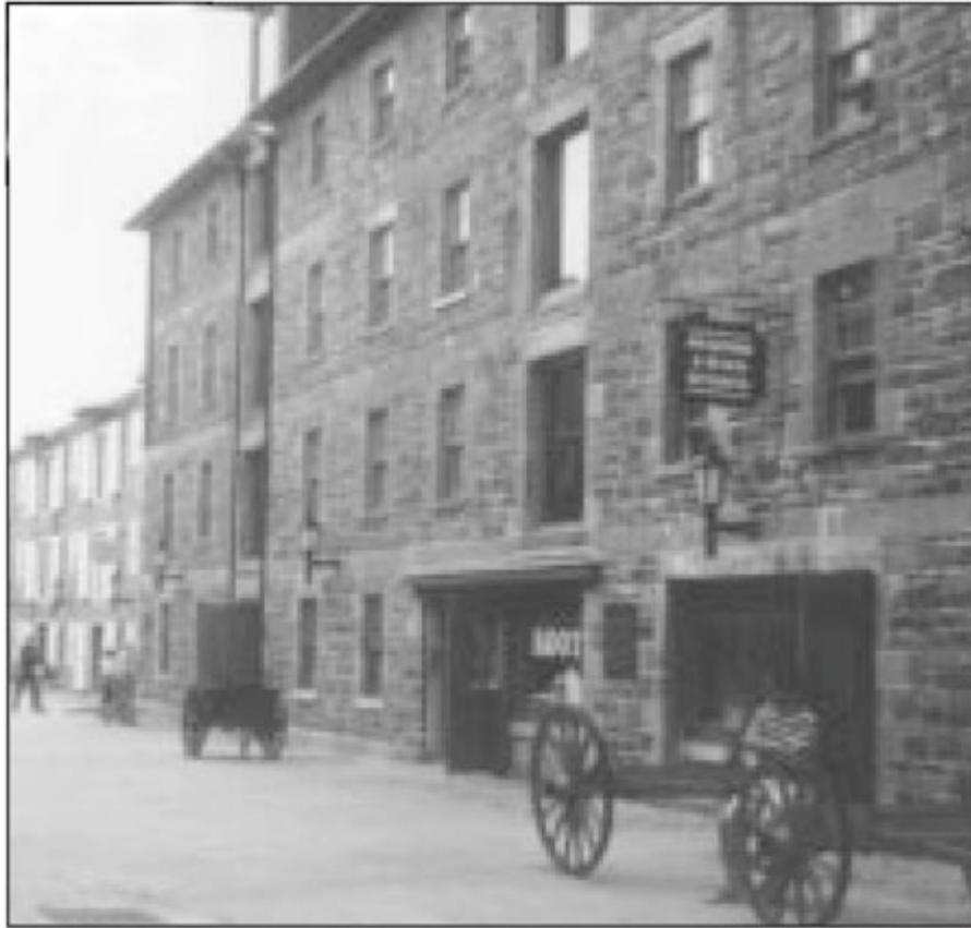
Figure 1. Massive masonry construction
